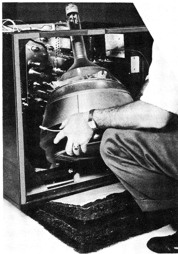
Fig. 75—Placing Kinescope in Cabinet
